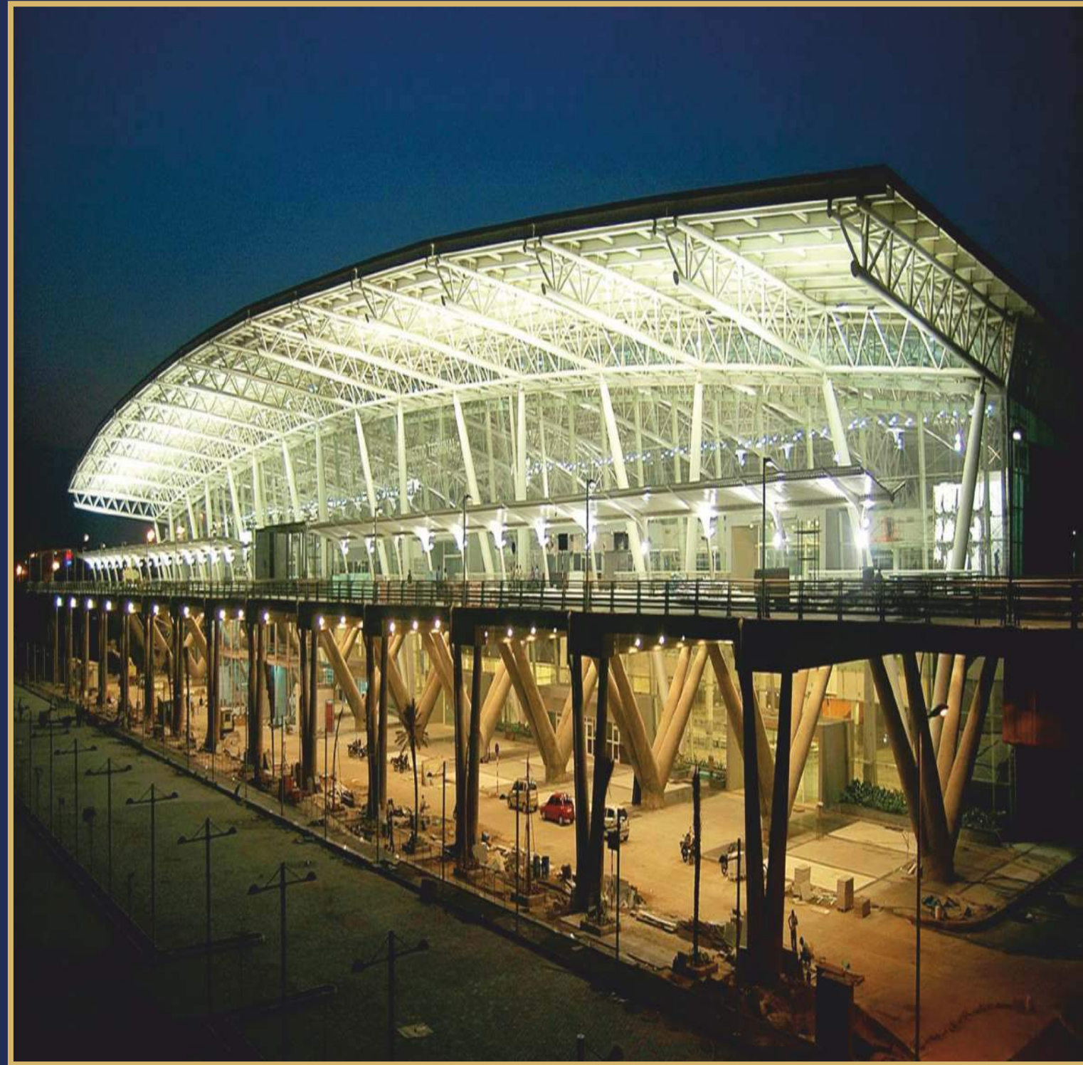
Chennai International Airport
